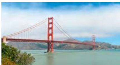
Golden Gate Bridge in San Francisco
